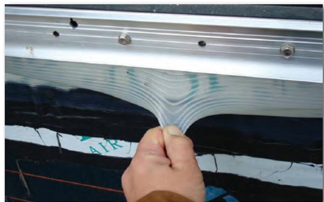
**The translucent silicone extrusion incorporated in the Proglaze ETA composition provides a “stressless” connection, eliminating movement as a design concern.**
