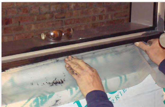
**Tremco’s Proglaze ETA Engineered Transition Assembly provides a tested, durable connection from the air barrier to the window assembly.**
