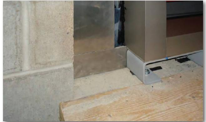
**Self-adhered membranes were not a viable solution to bridge joints in excess of ¼” to ½” or accommodate potential thermal or seismic movement.**
